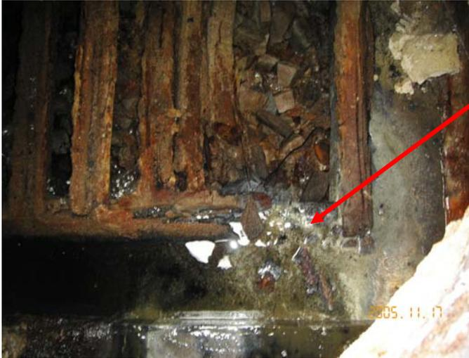
The main gutter is corroded here.
