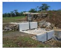
Filter bed using coral tip and coconut husk activated carbon
